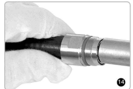
Flare the outer conductor, separate the outer conductor from the insulator.
